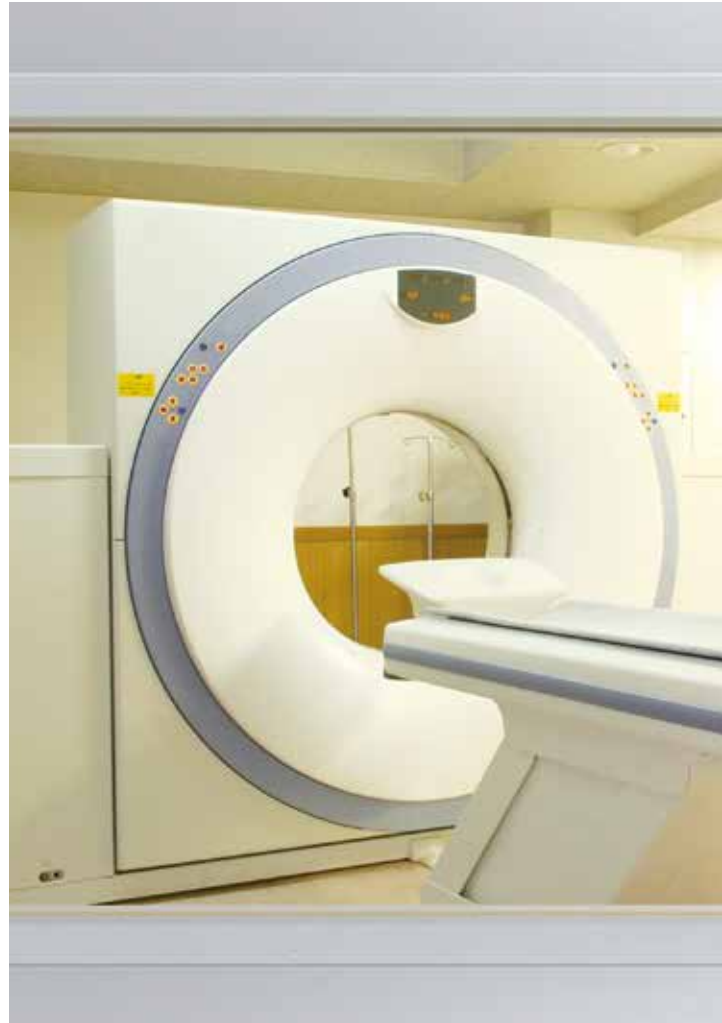
Viewing window for CT room
